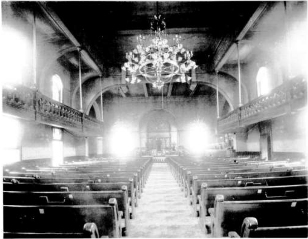
INTERIOR MAIN STREET METHODIST CHURCH.
